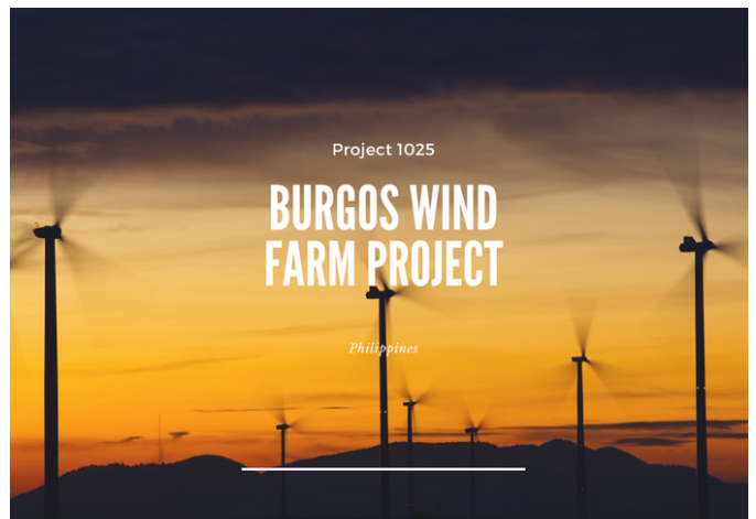
Project 1025: Wind Power in the Philippines
